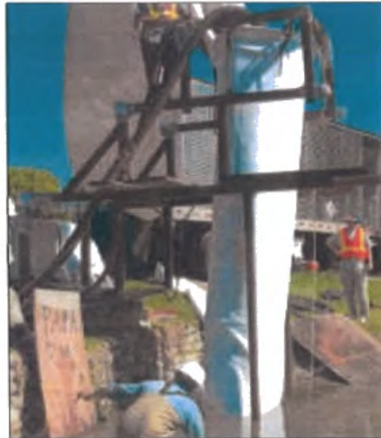
Subaqueous installation of CIPP into storm drain
