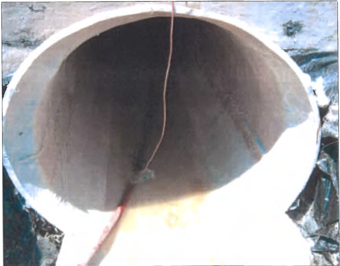
Finished outfall product at the headwall
