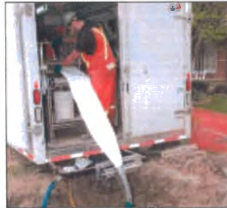
ASTM F1743 Pull & invert technology
