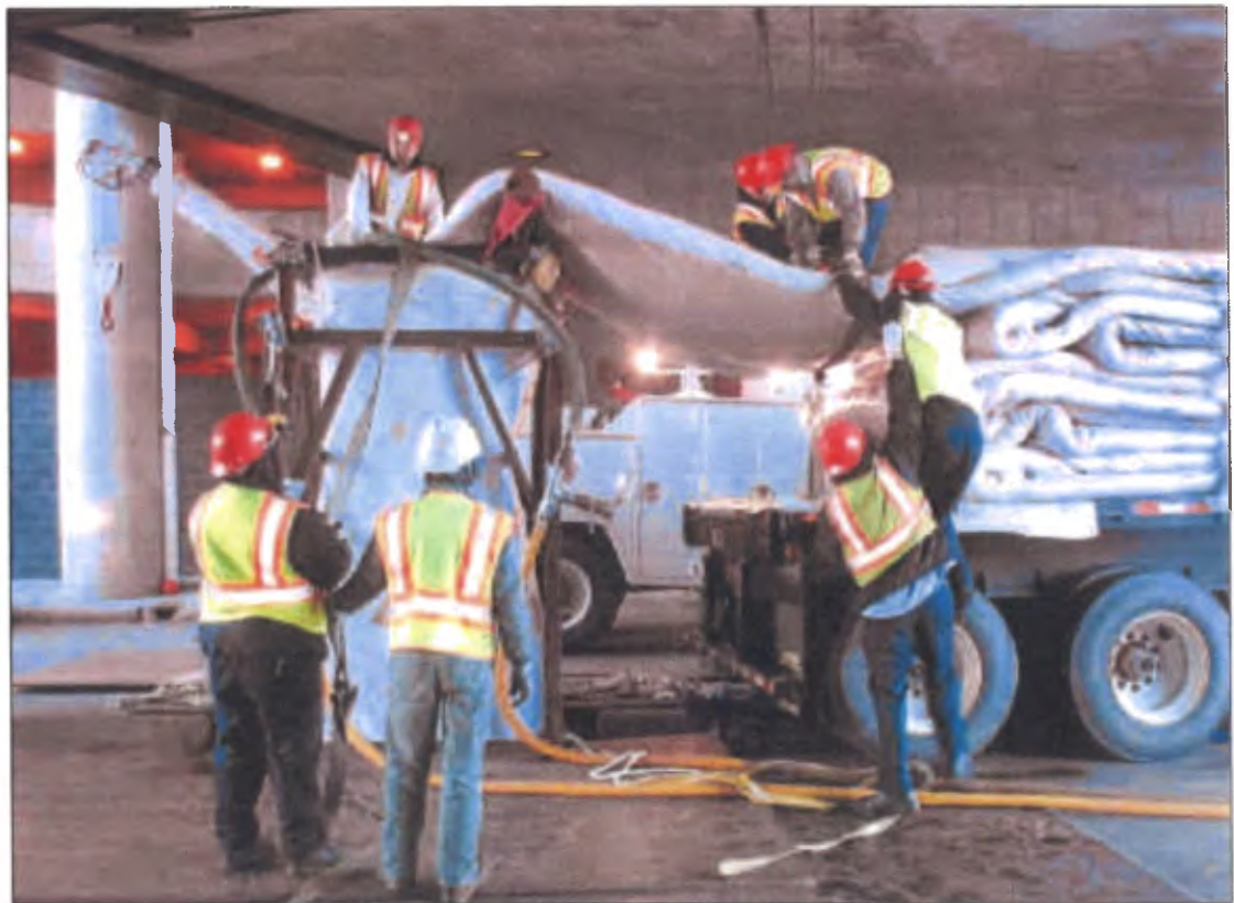
Rehabilitation of 900 feet of 72-inch sanitary trunk sewer at "The Joe"
