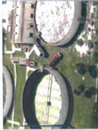
Cantilever pressure pipe rehabilitation at WWTP
