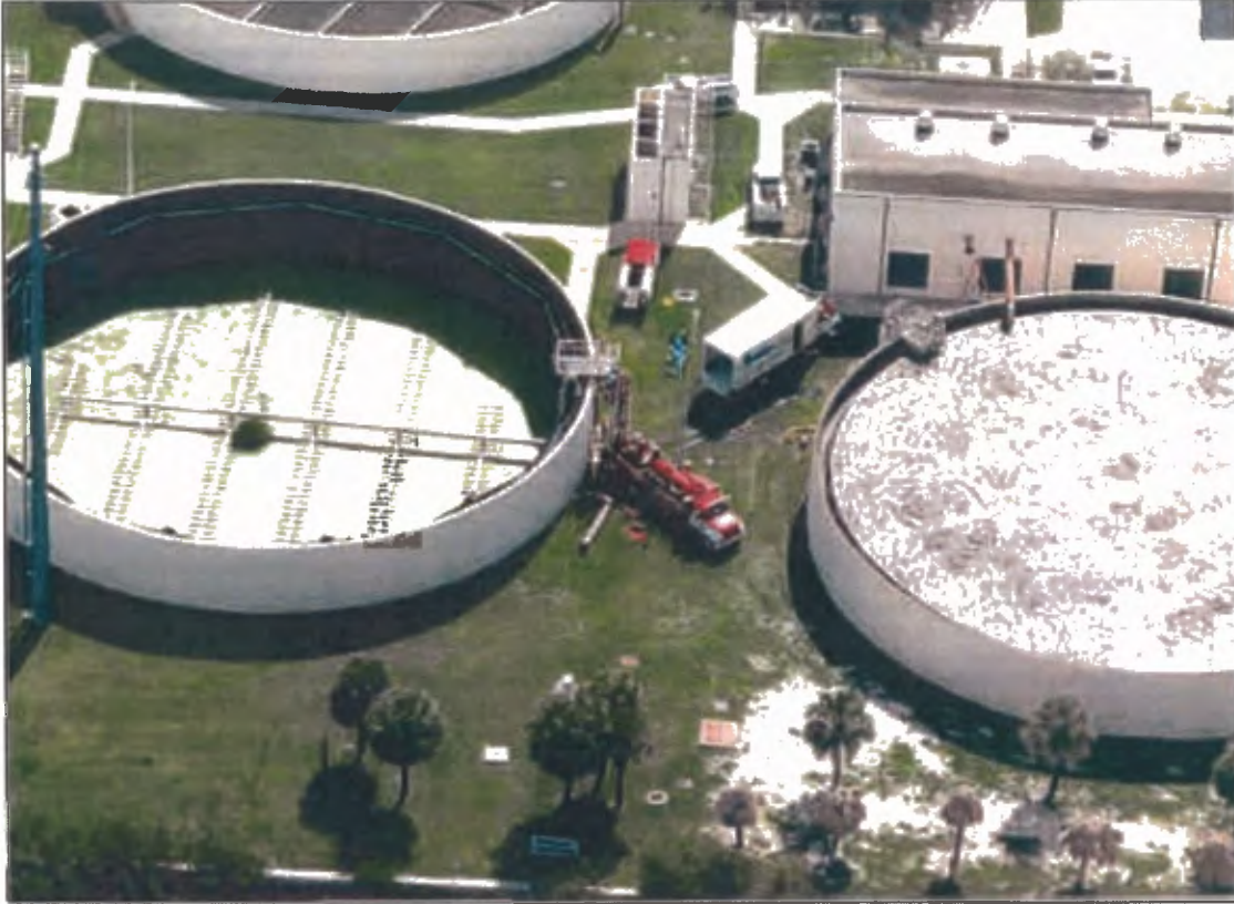
Clarifier pressure pipe rehabilitation at WWTP
