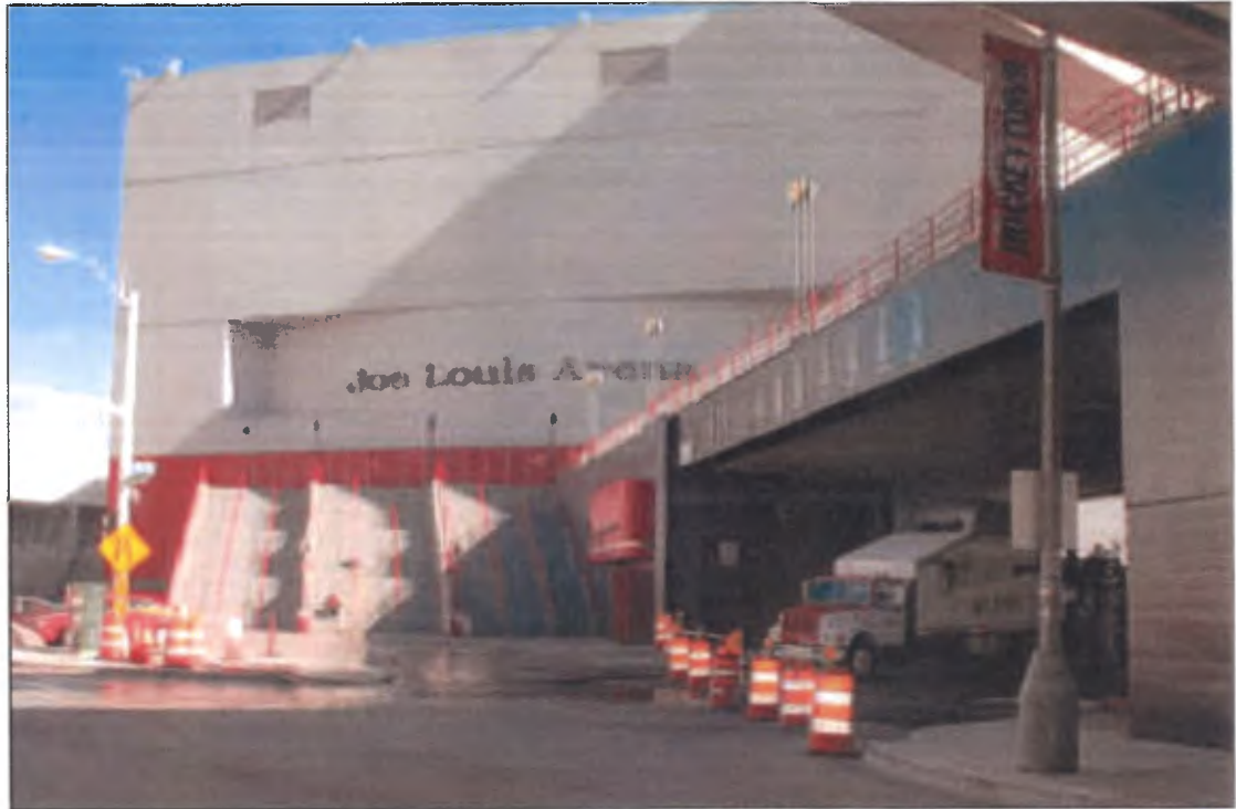
CIPP installation at Joe Louis Arena – Home of the Detroit Red Wings
