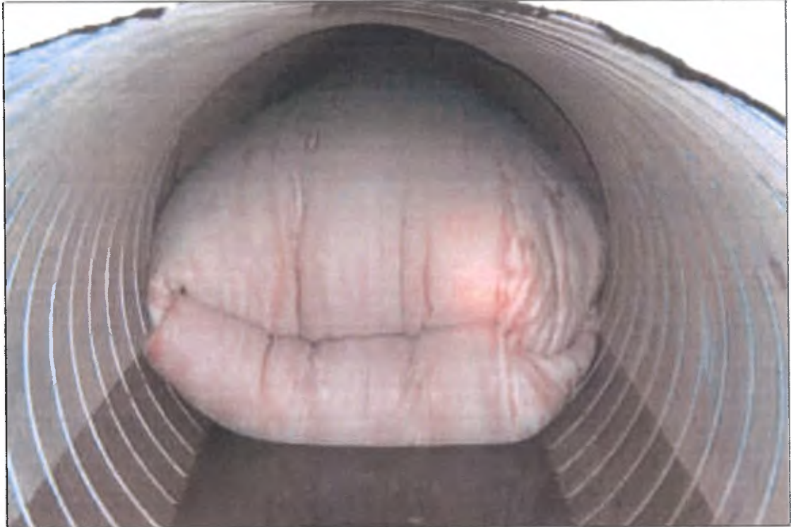
Frontal view of 60 inch diameter direct inversion
