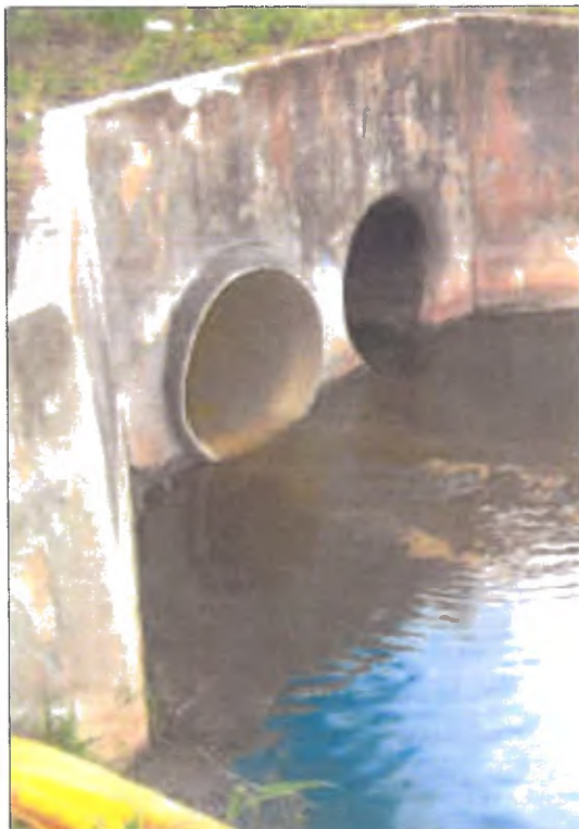
Trenchless renovation in storm drain application
