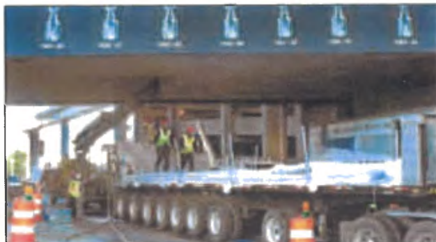
Large bore trenchless renovation in "tight quarters"
