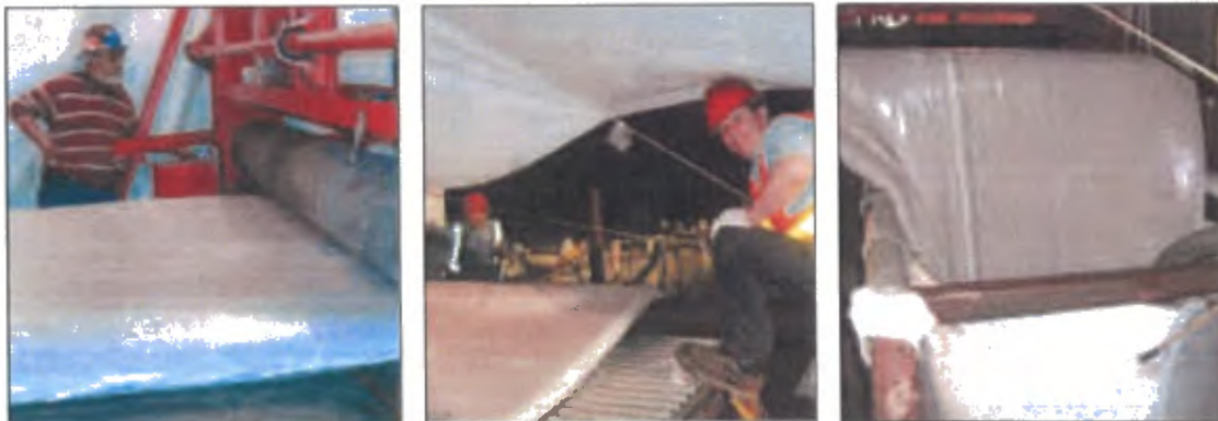
"Over the hole" wet out and installation of large bore circular, non-circular, and box culvert applications
