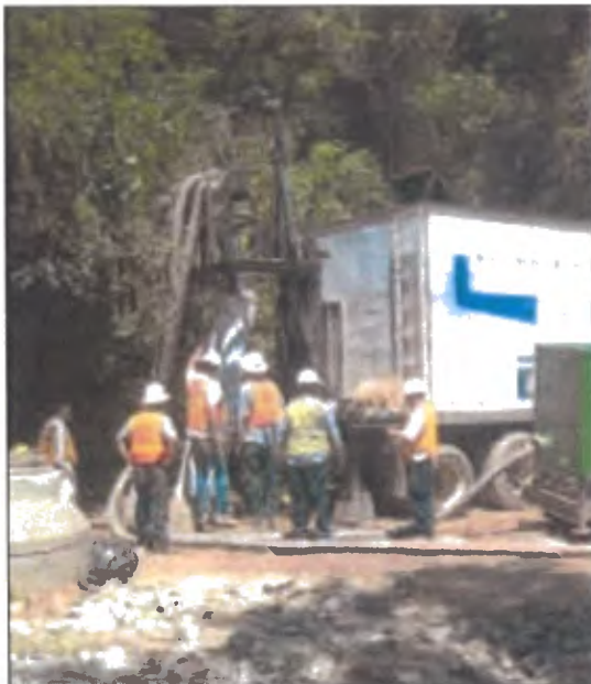
Easement installation of subdivision sewer rehab
