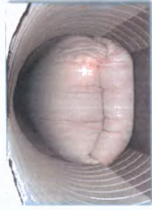
Frontal view of 60 inch diameter direct inversion
